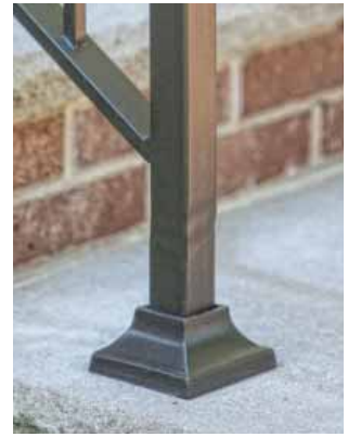
Detail of cover shoe to add aesthetics and protection to base of post
