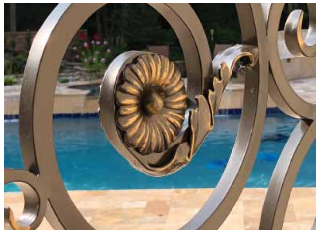
Detail of forged rosette and leaf for stair railing
