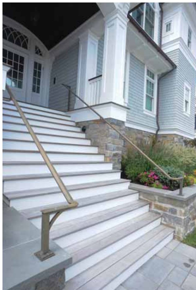
Solid bronze handrails meets code for stair railing
