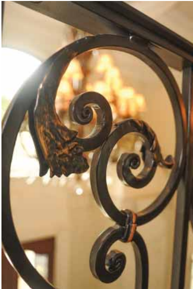
Close up of forged scroll detail for house railing
