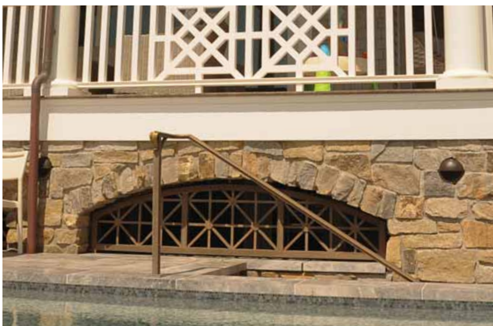
Powder-coated solid aircraft grade aluminum pool fence
