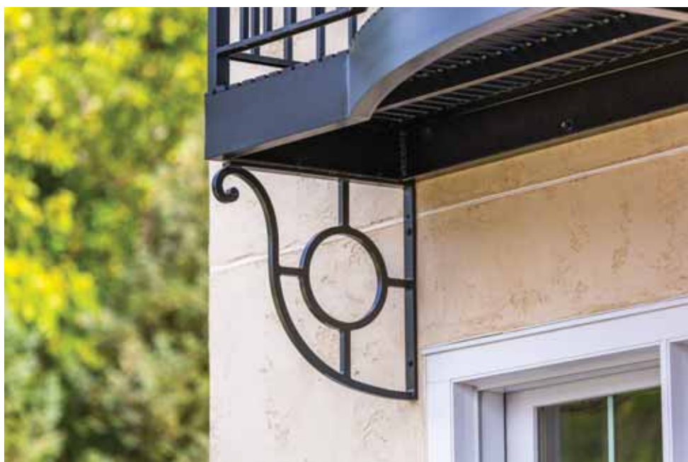
Brace detail for balcony and railing
