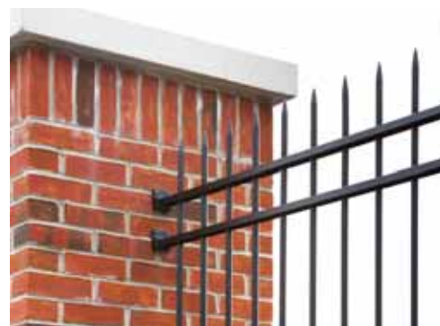
Left: Iron fence provides a safe and authentic barrier for today's commuters. Right: Custom forged pickets for authenticity.
