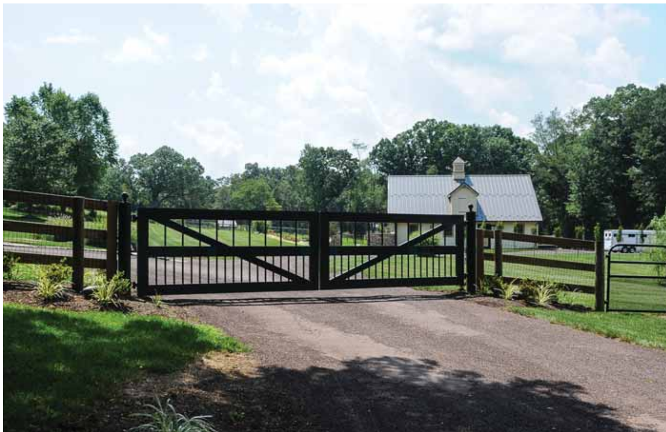
A simulated wood gate done in non-corrosive aluminum
