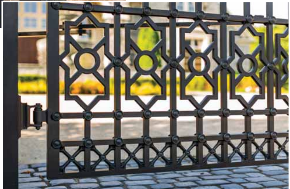
Close up of custom detail and forged rosettes
