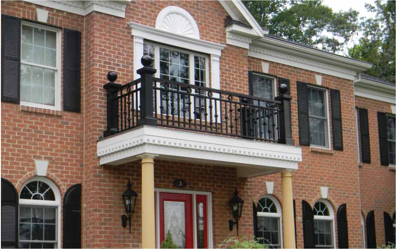
Solid aluminum railing with 6" Hampton posts
