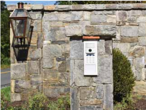
The mobotix keypad to integrate into smart home system to operate gate openers
