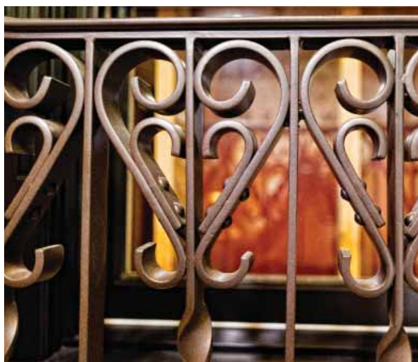
Close-up of hand-forged scrolls and rivets
