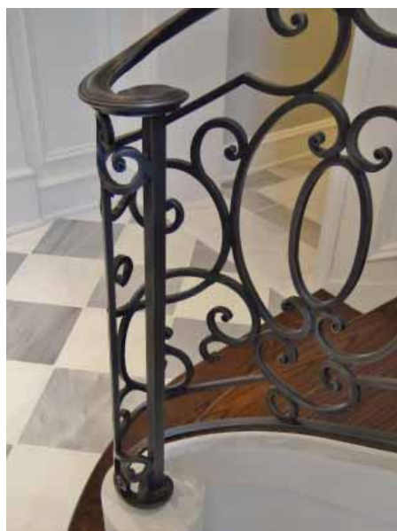
Custom forged iron volute for stair handrail with antique tarnish
