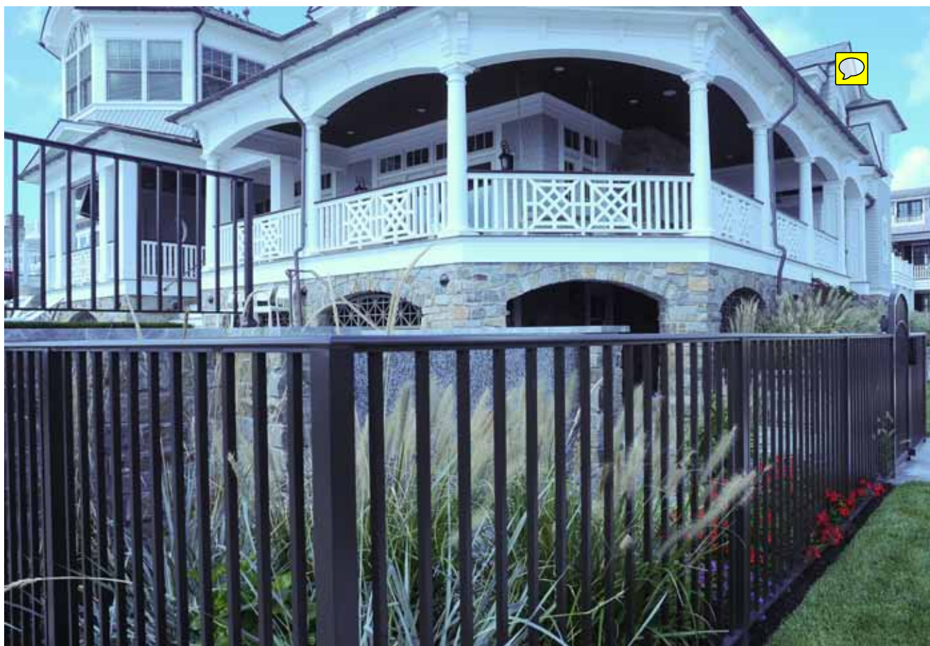
Powder-coated solid aircraft grade aluminum pool fence
