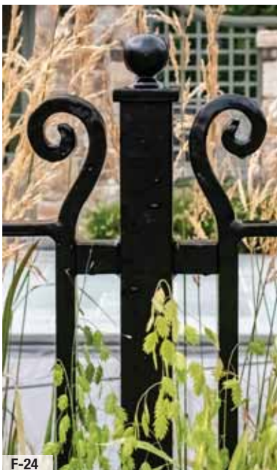
Hand forged scrolls flanking fence post.
