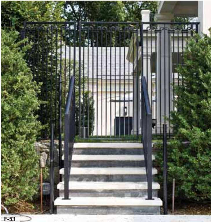
Modern Pool Fence and gate.
