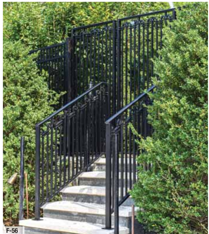
Pool fence and railing that meets all safety requirements beautifully.
