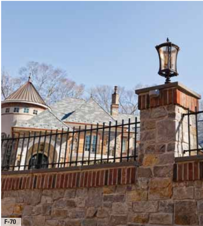
Saratoga fence with classic pickets adorns the top of a retaining wall
