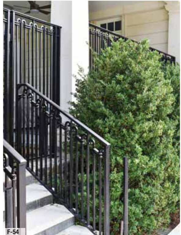
Railing design enhances pool fence design.
