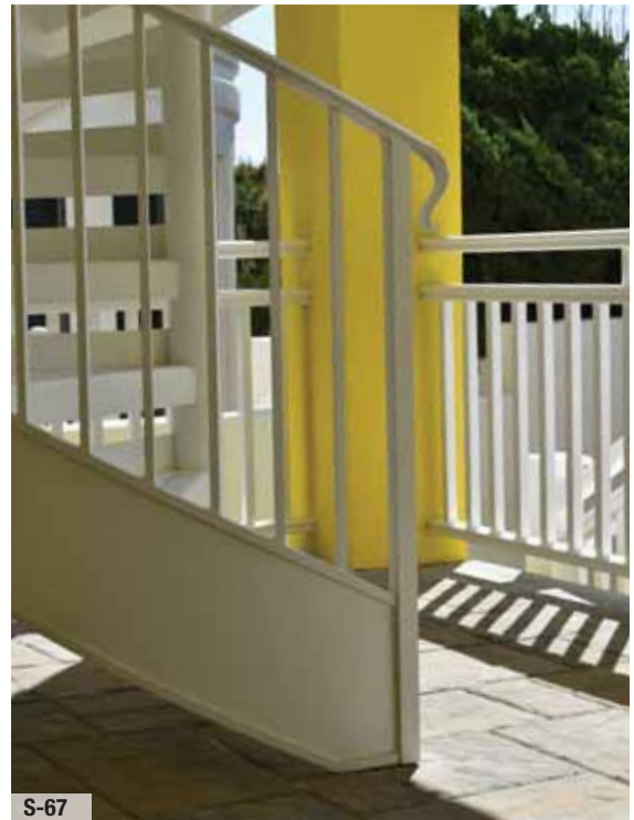
Classical railing design with outer skirt structure.
