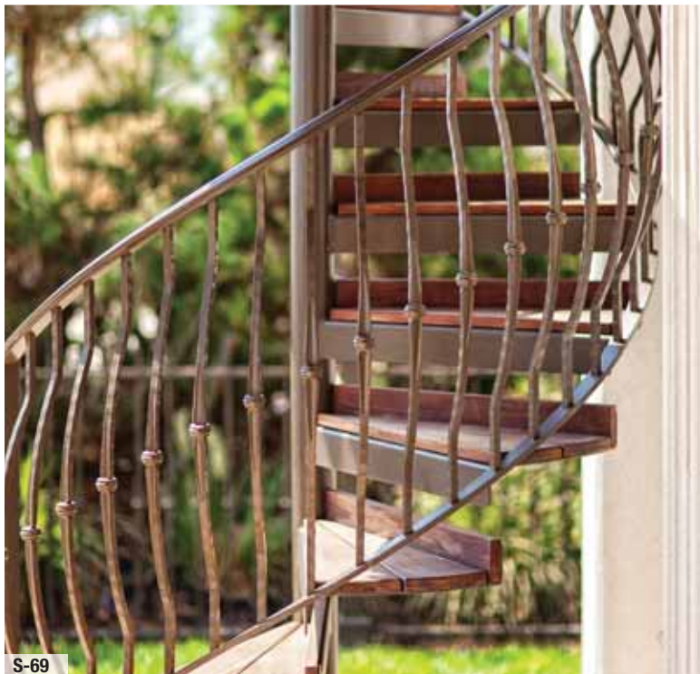
Railing attached directly to the treads.
