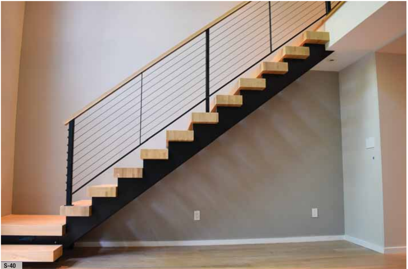
Modern stair with cable rail and a block wood caprail.
