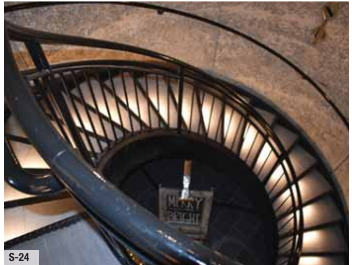
Tower stair topview
