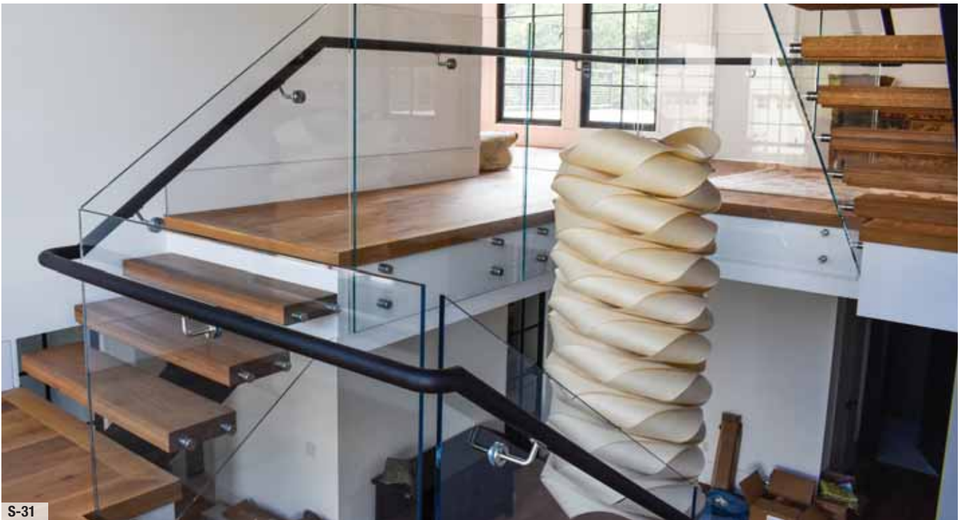
Mono-stringer staircase with glass railing design.
