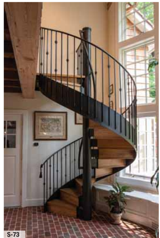
Exposed picket design along the outside of the spiral ribbon.
