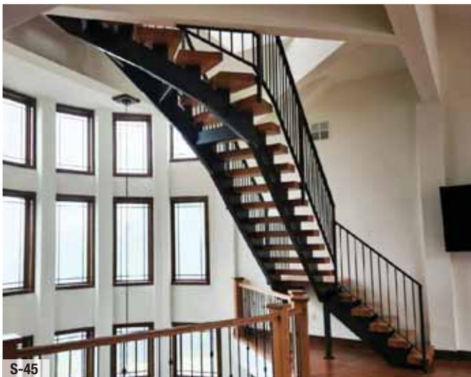
Double tube stringer structure detail.
