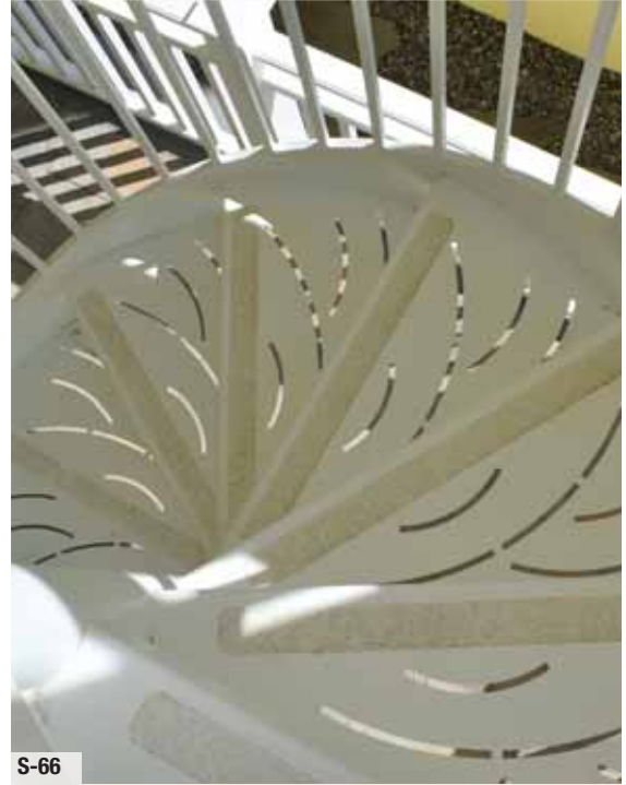
Custom laser cut wave treads.
