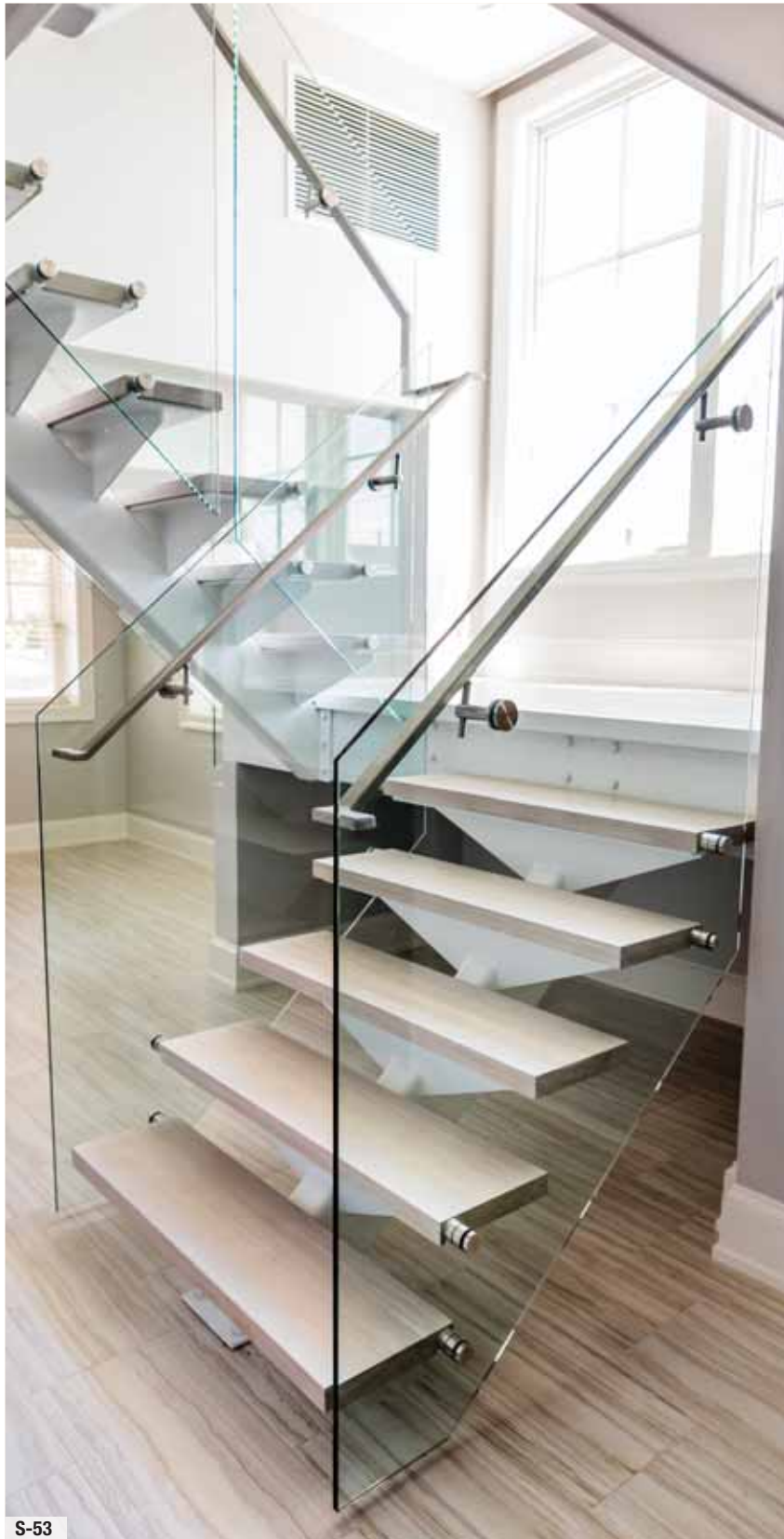
The beauty of glass railing on a landing and switch back stairs
