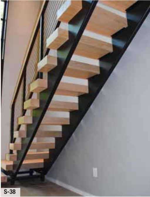
Double sawtooth stair stringers
