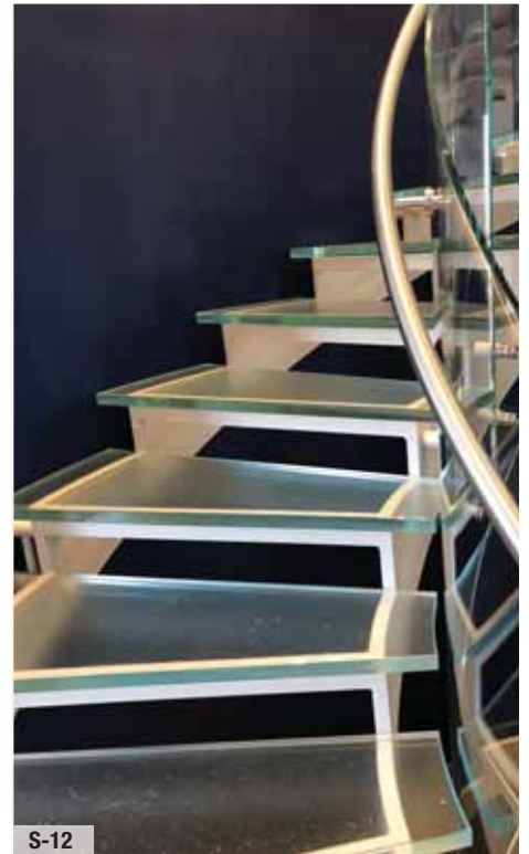
Translucent glass treads on curved stair
