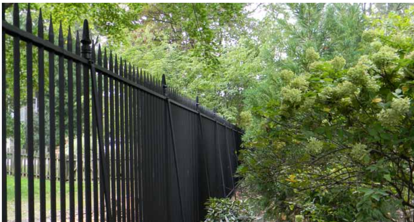
The classic braces on a Villanova fence add stability
