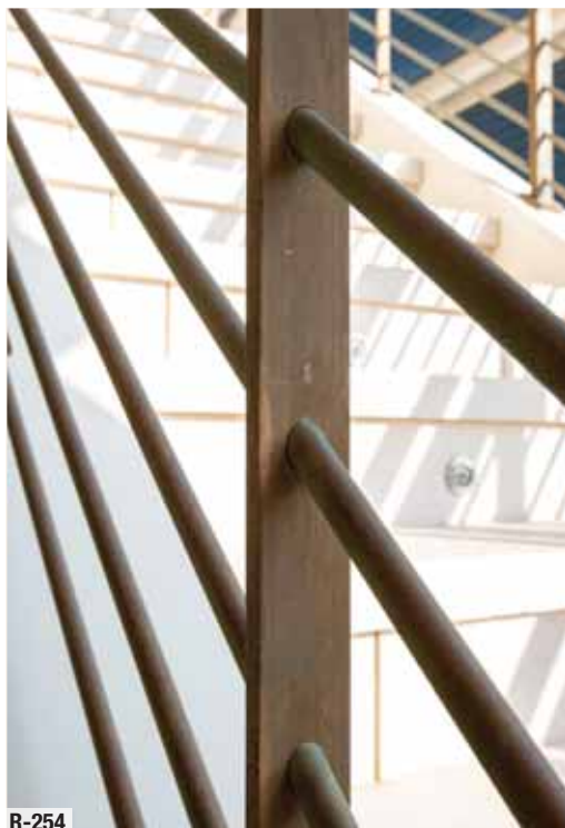
Innovative post/railing connections on bronze railings.
