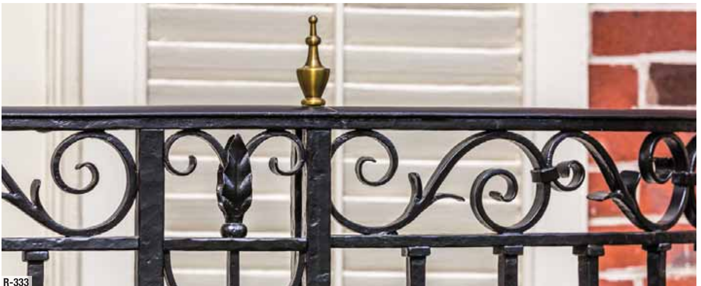
Bronze finial restored above scrollwork restoration.
